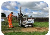
Ground Investigation (GI) work was a large part of the technical preparatory work, with over 300+ samples conducted between July and September 2023. Laboratory testing and data factual reports of the results of the GI were complete in November 2023. This information is a key component in developing the detail design of the walls, ensuring we have undertaken necessary technical due diligence to confirm what we propose will work and remain functional for many years to come.
